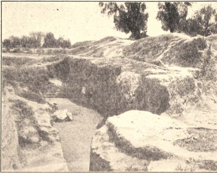
Fig. 4. Kanishka-chaitya after excavation.
